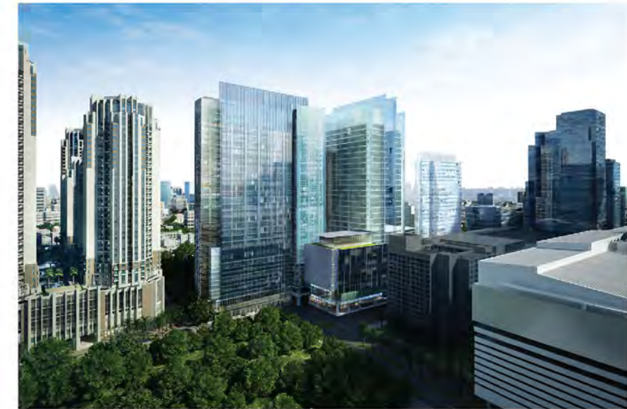
- Photo of The Ninth Tower Grand Phra Ram 9 Office Building Project when completed -
