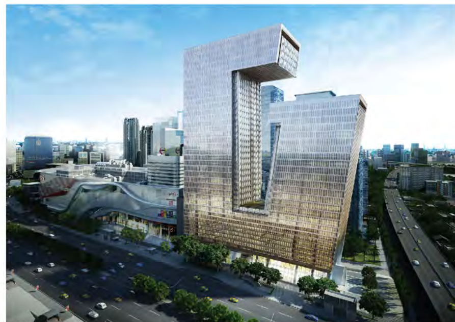
- Photo of G Land Tower Grand Phra Ram 9 when completed -
